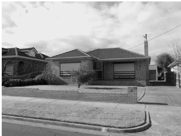
FIGURE 1. The stereotypical image of the nonmigrant “cream-brick-veneer house,” 2012. Photograph by Iris Levin.
