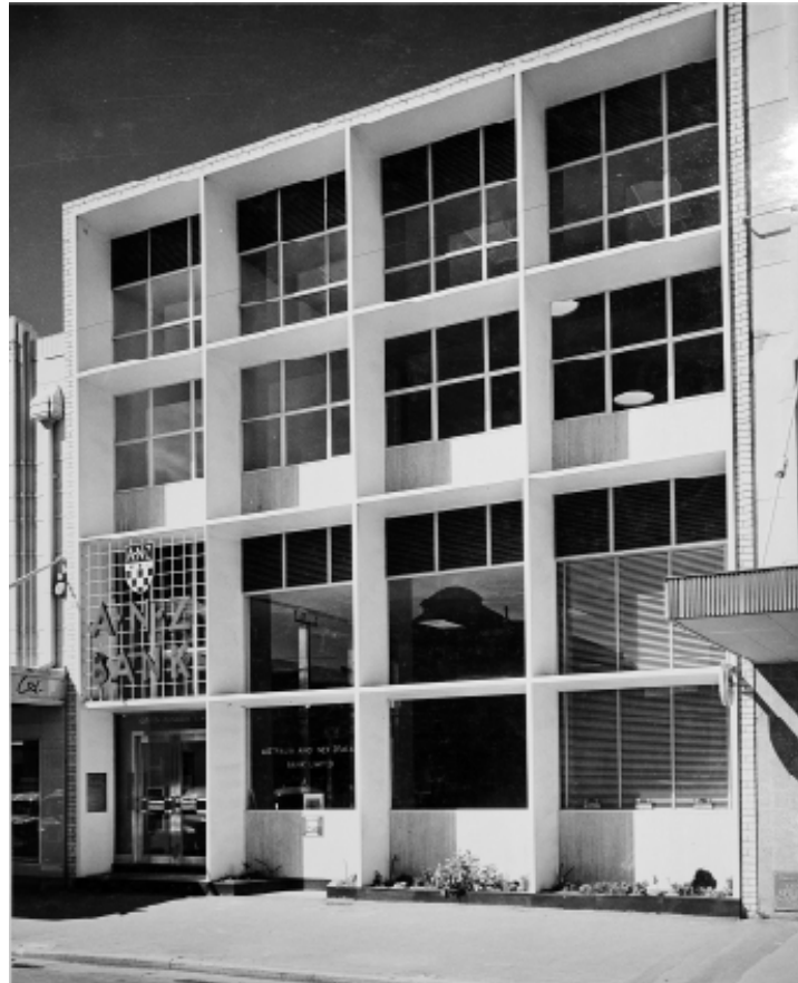
Figure 8: ANZ Bank (c. 1955), Flinders Street, Adelaide City. (Source: Jack H McConnell Collection, Architecture Museum, University of South Australia, S270/1/1)
