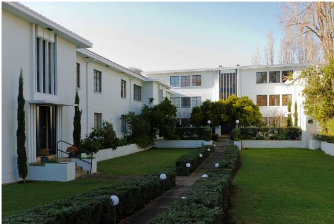
Figure 3: Deepacres Apartments (1942), Melbourne Street, North Adelaide. (Photograph: Paul Wallace)
